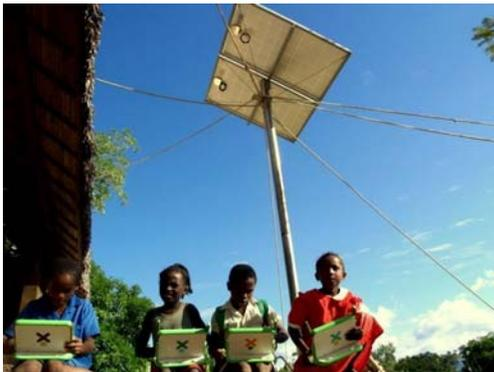
Being close to the Equator and having a clear sky for most of the year, Nosy Komba is the perfect place for power generation with solar panels. So, in 2011, we mounted **two photovoltaic installations with four solar panels of 220 W, providing electrical power to the school campus and the community farm.** The electricity generated by these installations is mostly used for lighting and allows evening classes.
